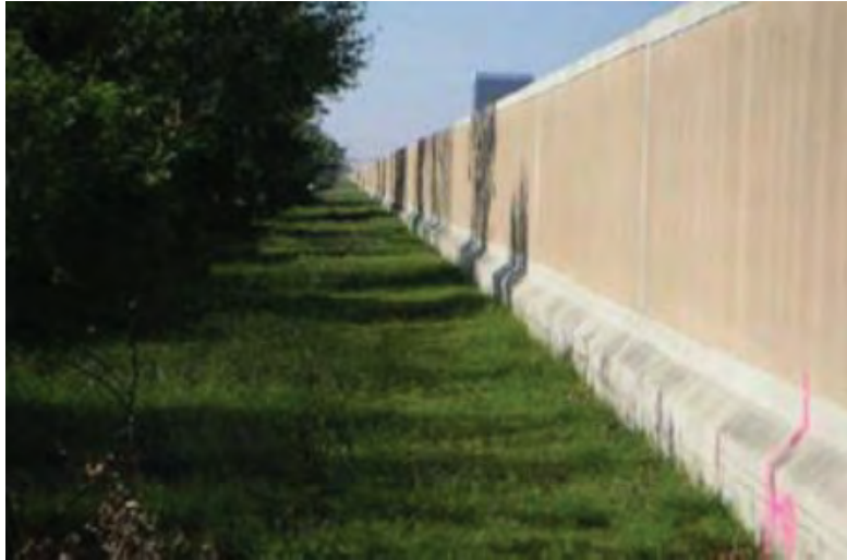
Figure 49: Typical Floodwall Construction along the 17th Street Canal in New Orleans
