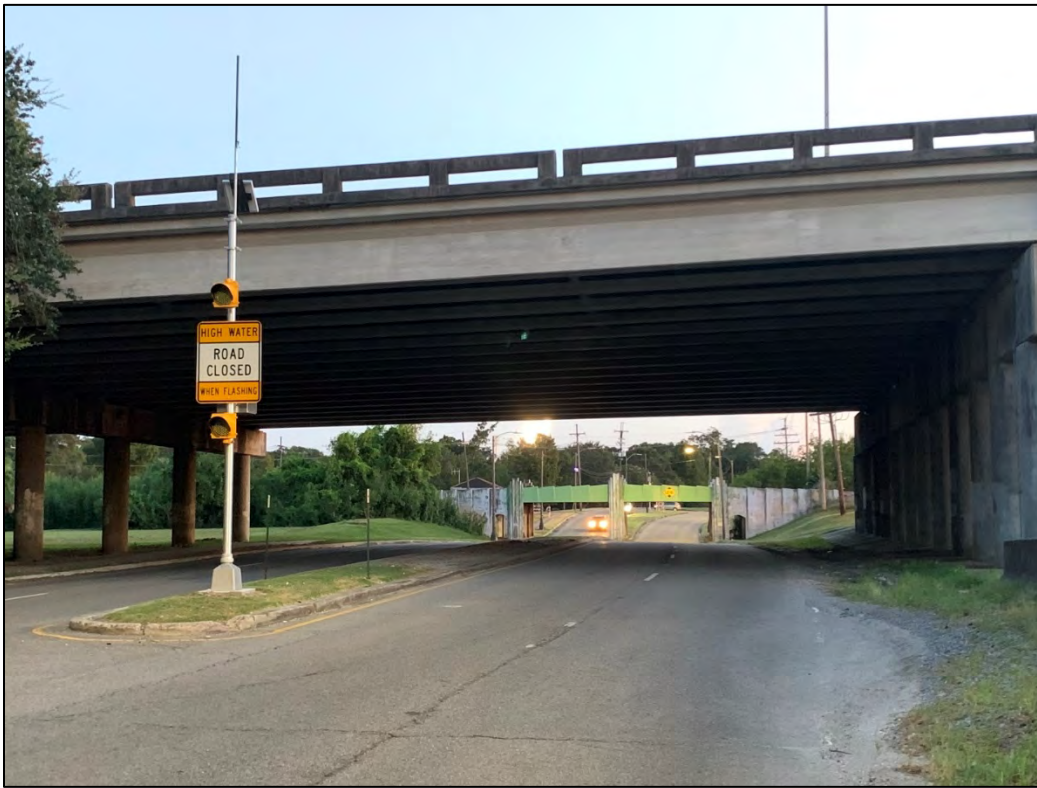
Figure 52: Automated Flood Warning System on Marconi Drive
