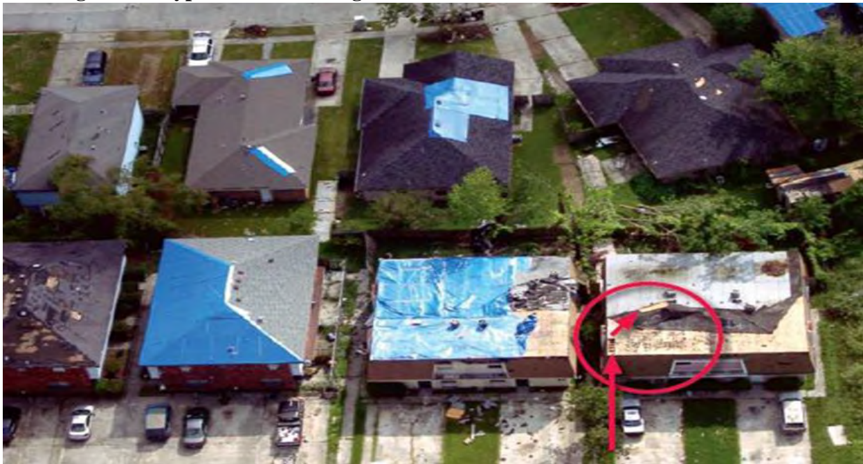
Figure 28: Typical Wind Damage to Residential Structures – Hurricane Katrina
