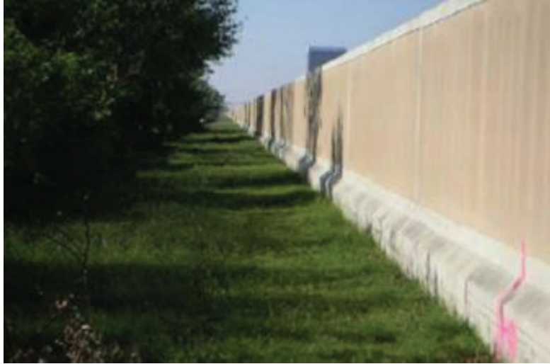
Figure 48: Typical Floodwall Construction along the 17th Street Canal in New Orleans
