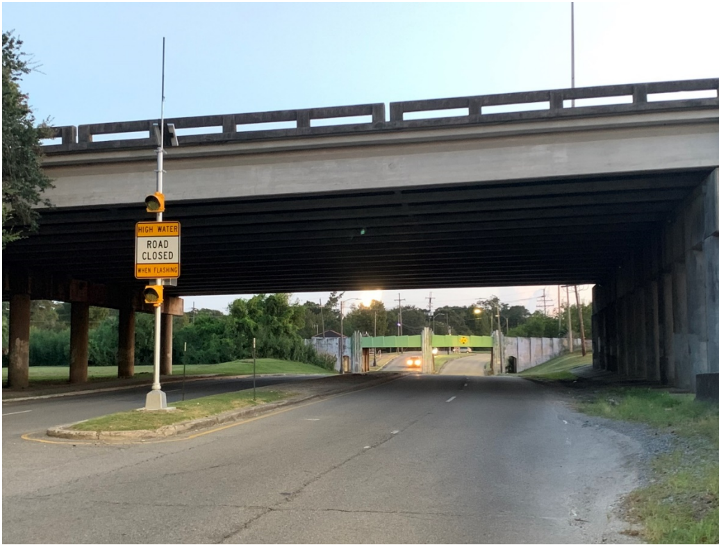
Figure 51: Automated Flood Warning System on Marconi Drive
